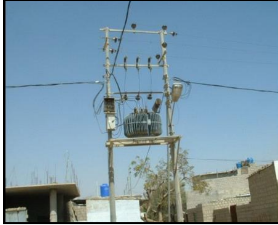
Figure 2. After Installation of ABC
